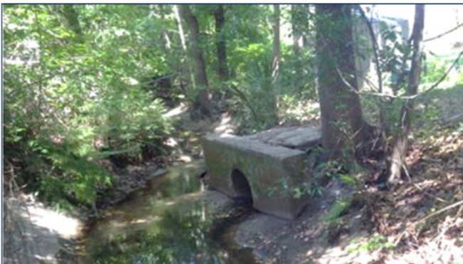
Major Outfall, City of Jacksonville Public Works
