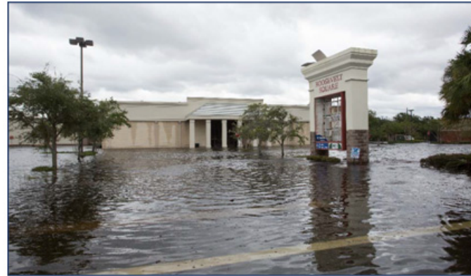
Hurricane Irma – Roosevelt Square Shopping Center, September 11, 2017
